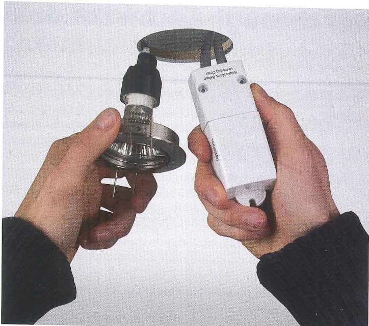
This Timeguard ZV900 is small, inexpensive, easy to install, slips neatly through a standard 50mm ceiling aperture and you only need one per switching circuit.
